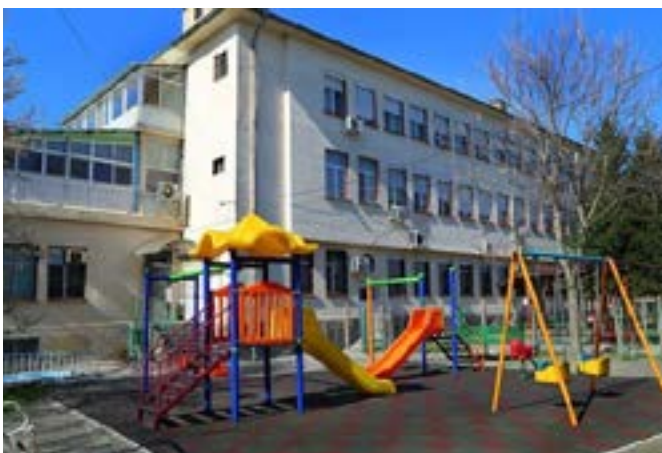
Image 2: The center in Debelets, in the same building as the former Home for Medico-Social Care for Children. 82
